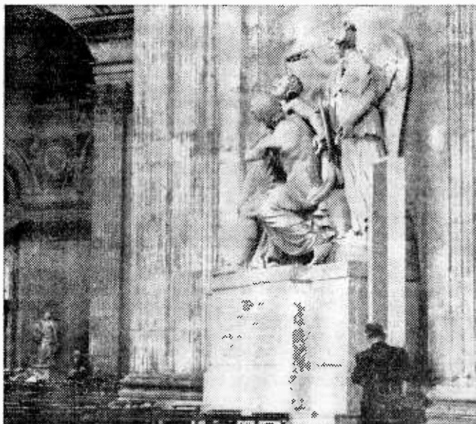
An STC engineer positions an 8 ft. column loudspeaker in St. Paul's Cathedral during recent acoustic tests.
